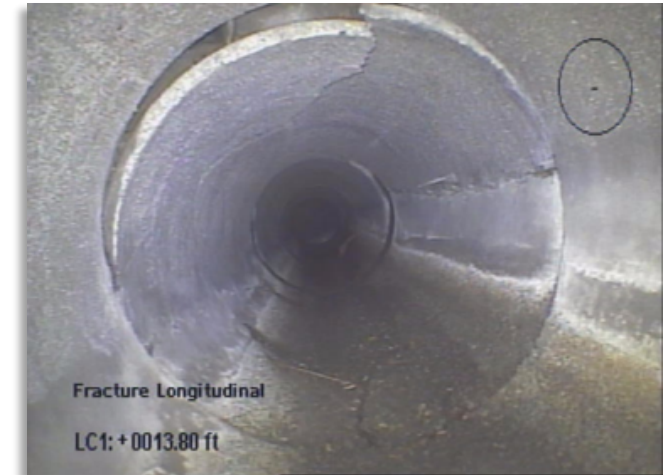
View inside stormwater Pipe
