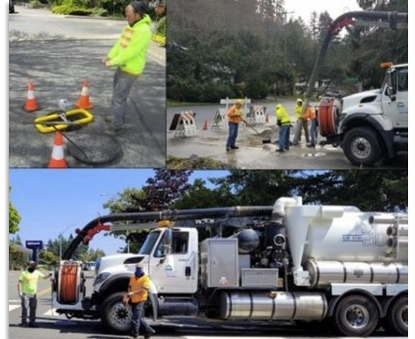
Wastewater Crews In-Action
